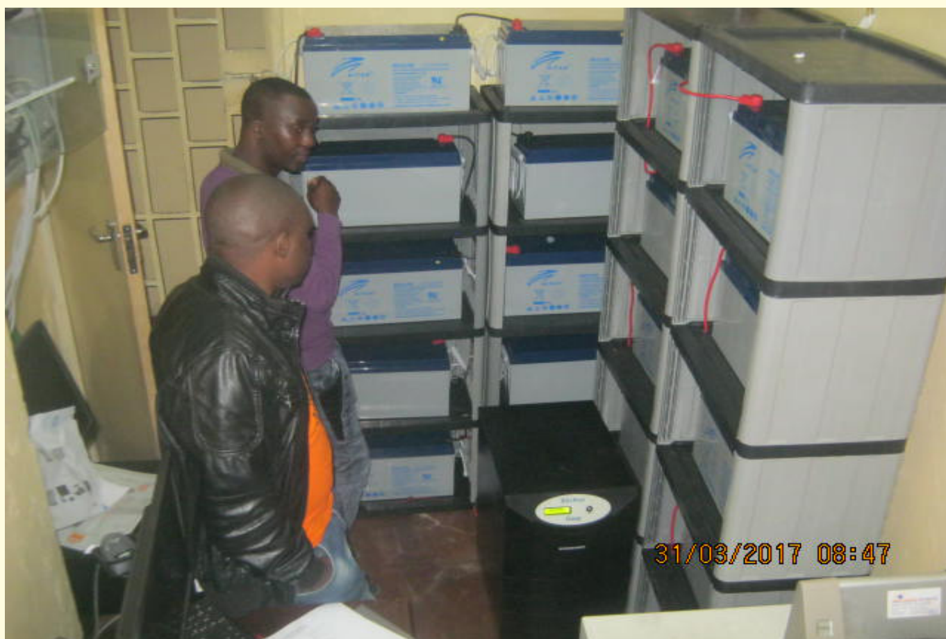
Fig. - Part of the fully installed UPS Equipment at Monze RTSA station
