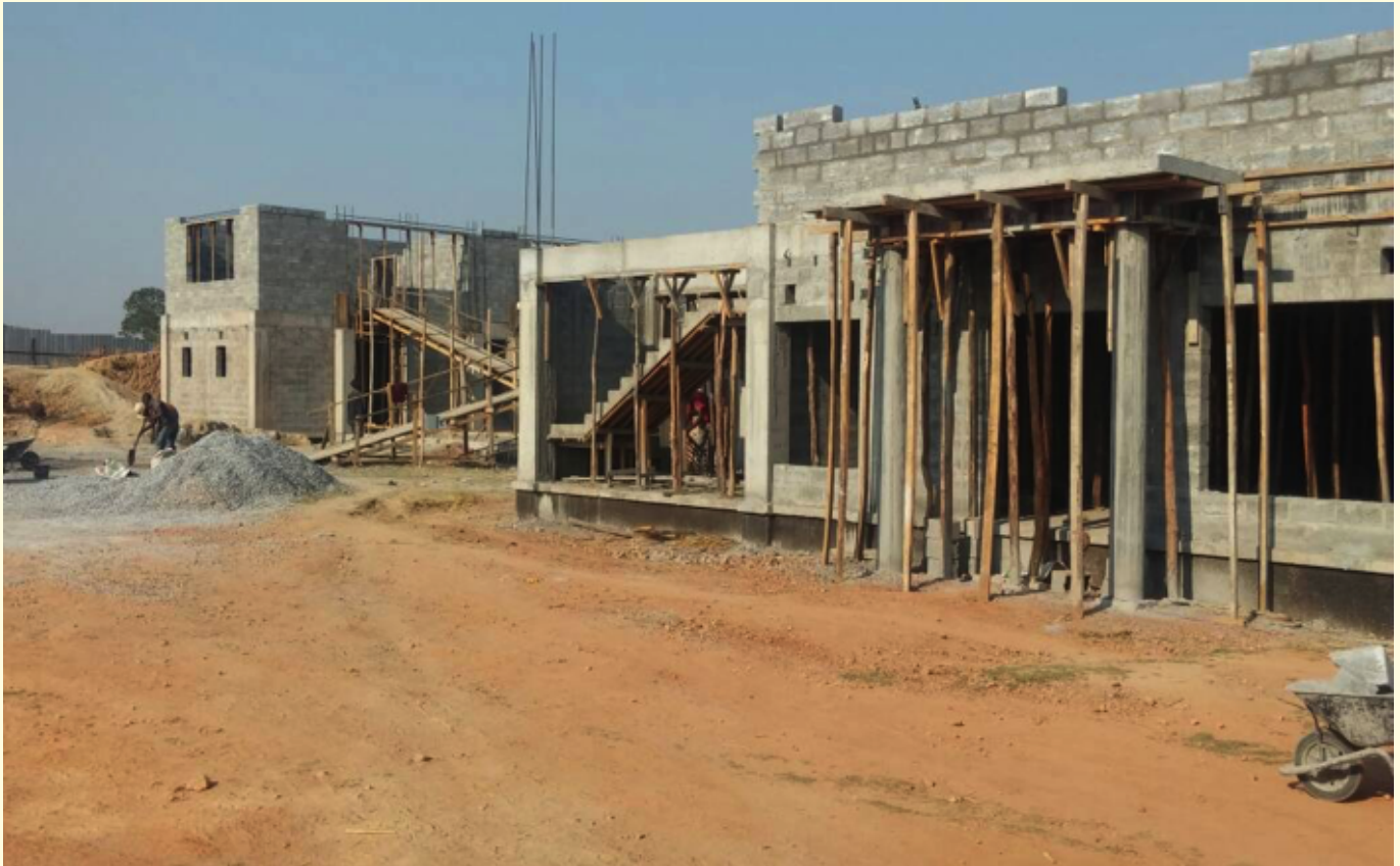
Construction of Motor Vehicle Inspection Centre in Luanshya – substructure, blockwork & columns
