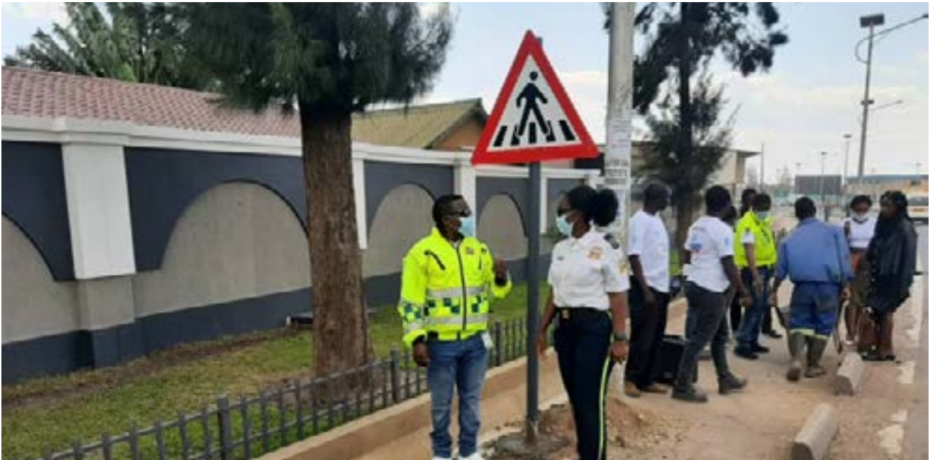
Figure 4: Installation of Road Signs
